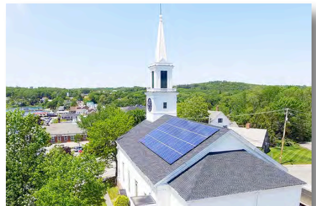
Source: U.S. Department of Energy
