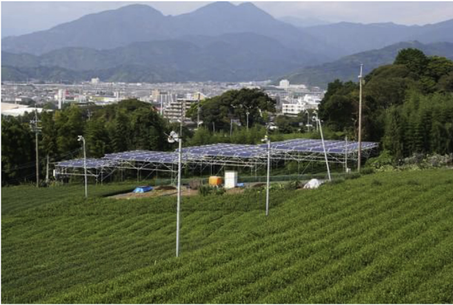
Fig. 1. AVS example (An AVS on a Japanese tea farm plot in Shizuoka prefecture, Japan). Reference: Zenkoku Einogata Hatsuden Kyokai (2017) http://farmsolar.or.jp/ .
