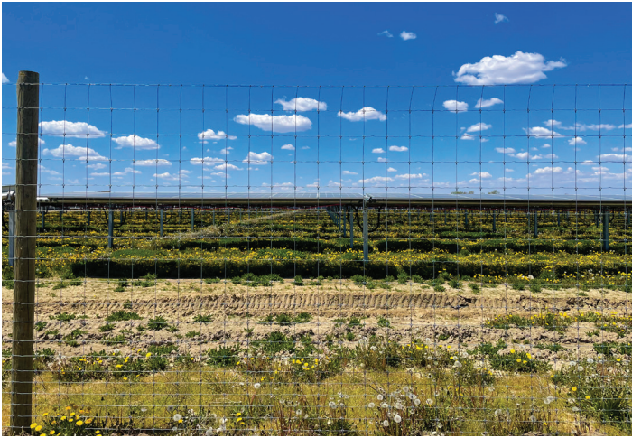
Figure 10. Scorecard-compliant pollinator habitat in its first season on preserved farmland at the Assembly Solar facility in Shiawassee County, Michigan. People who toured the facility were surprised to only see dandelions and not wildflowers. (Photo by Sharlissa Moore, May 2021. Adjusted in Adobe Lightroom.)
