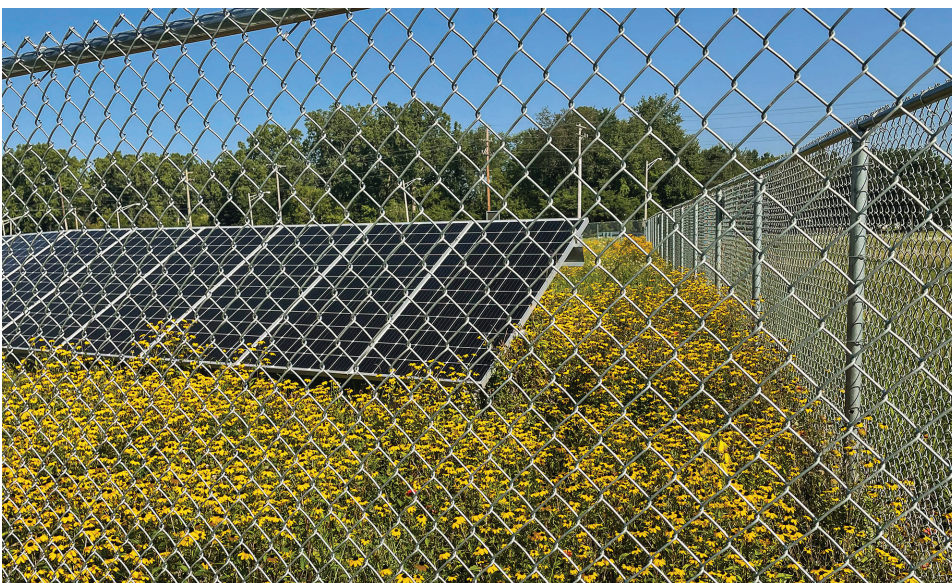
Figure 14. 300 kW community solar power plant built on a landfill, with pollinator habitat that is still establishing, in a residential neighborhood. No other development options were available for this site. East Lansing, Michigan. (Photo by Sharlissa Moore, August 2021. Adjusted in Adobe Lightroom)
