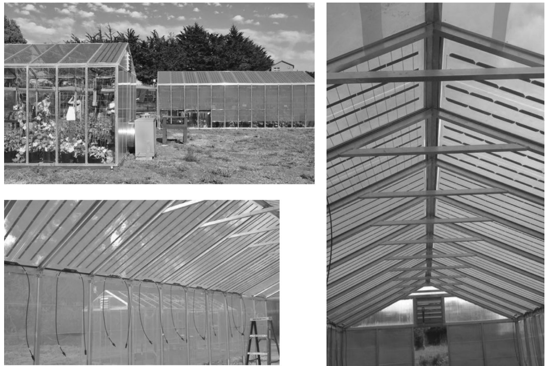
Figure 2. Glasshouse constructed with Wavelength Selective Photovoltaic (WSPV) panels, at the University of California Santa Cruz Arboretum. The WSPVs consist of polymethyl methacrylate (PMMA) plastic embedded with luminescent perylene red dye. The electricity generated by narrow photovoltaic strips (black lines in red panels) powers the operation of the glasshouse fans, microclimatic monitoring sensors, and data loggers. Photographs by Glenn Alers.
