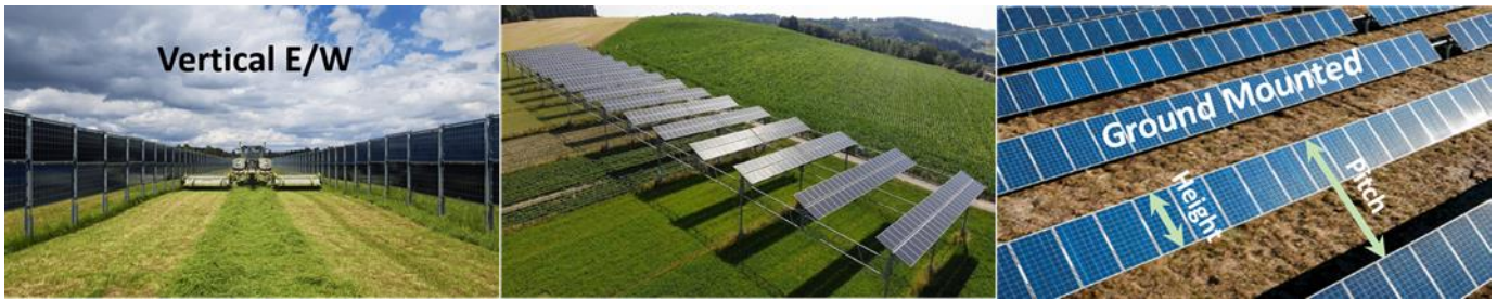
Figure 1. a) Vertical East-West (E/W) faced bifacial agrivoltaics (AV) farm [26], b) North south (N/S) faced agrivoltaics (AV) farm (source: BayWa r.e.) [12]. c) A typical ground mounted photovoltaic (GMPV) system with pitch and height labelled.
