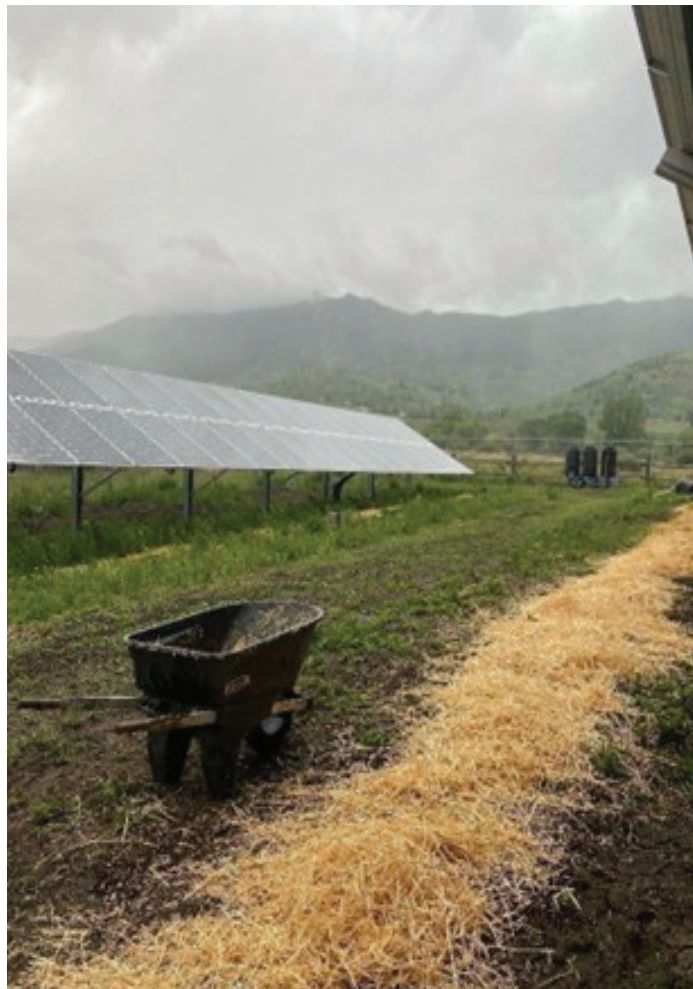
Planting in progress at the NCAT solar array. Photo: AgriSolar Clearinghouse
