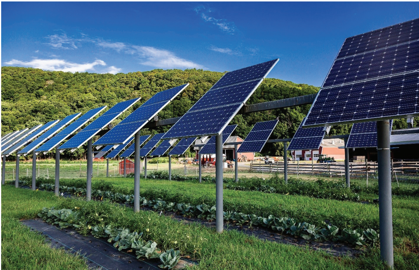
Agrivoltaic project at University of Massachusetts Crop and Animal Research and Education Farm. Photo: AgriSolar Clearinghouse
