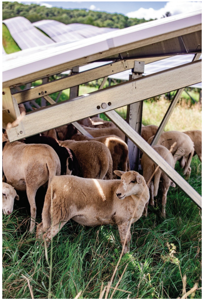
Single-axis tracking system at Jack's Solar Garden. Photo: AgriSolar Clearinghouse
