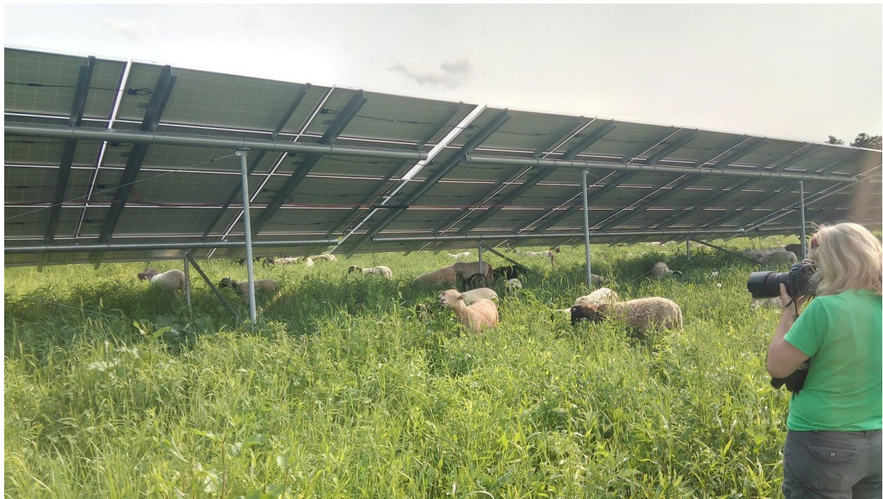
Figure S-6: The construction footprint of solar is a very small fraction of the solar installation – 0.2% to 2%. Sheep can graze almost everywhere else, including under the panels. Photo courtesy of The American Solar Grazing Association, with permission
