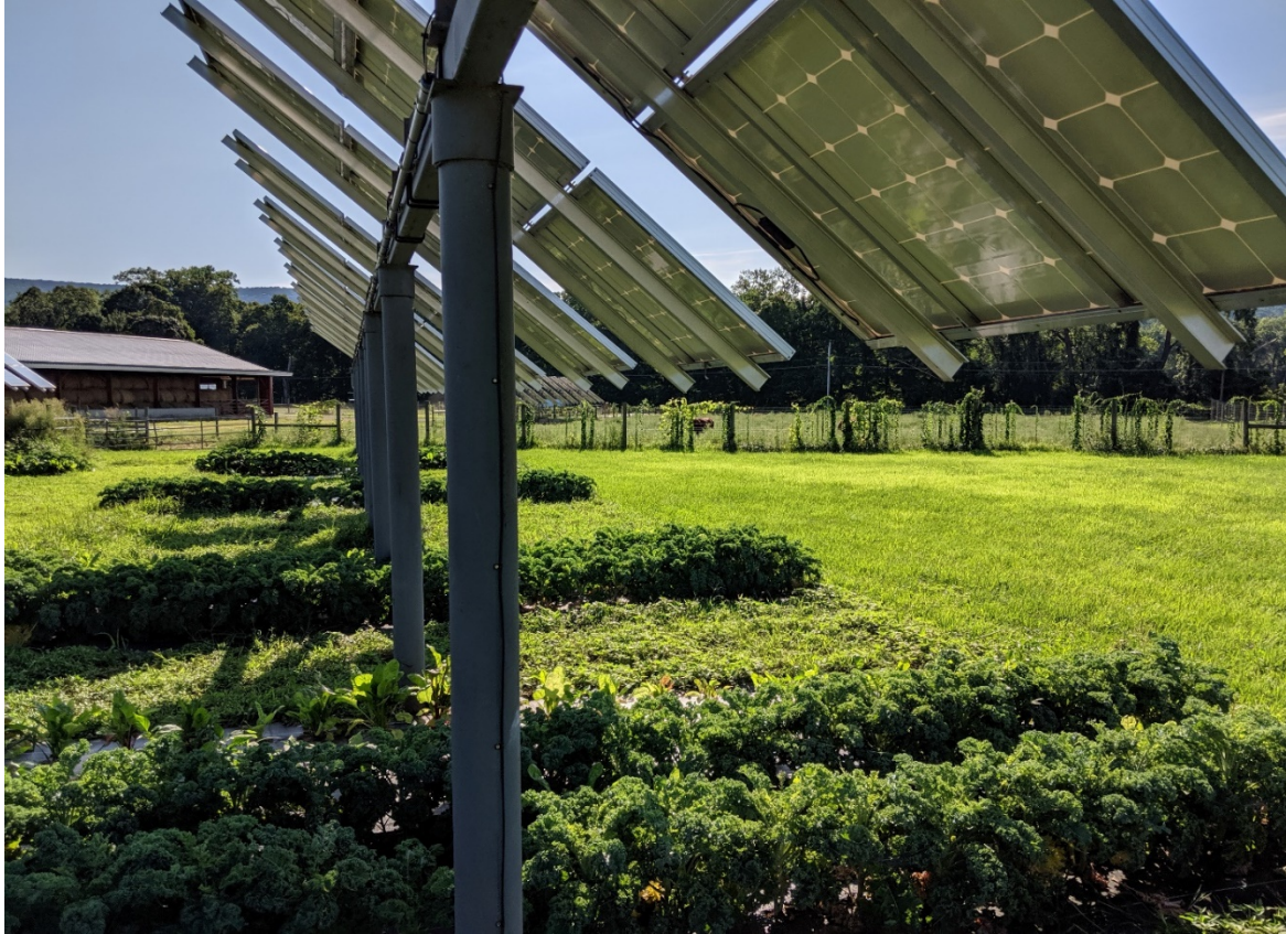
Figure II-2: Raised solar PV at the University of Massachusetts to allow for cultivation under the panels, showing post-driven, panel-mounting structure.
