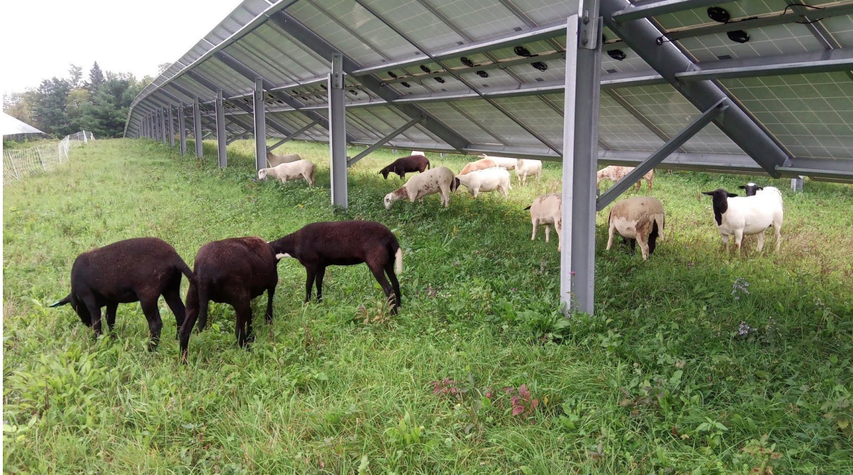
Figure II-1: A Ground mounted solar installation, showing small construction footprint; the panels also provide shade. Source: The American Solar Grazing Association ; with permission.
