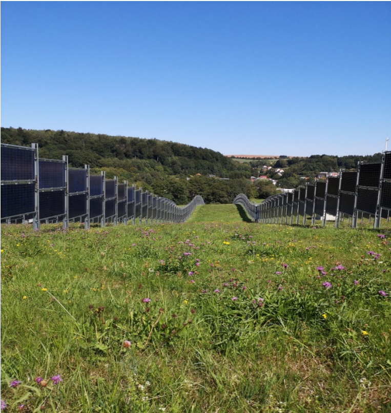
Figure II-4: Vertical, East-West solar panel configuration
