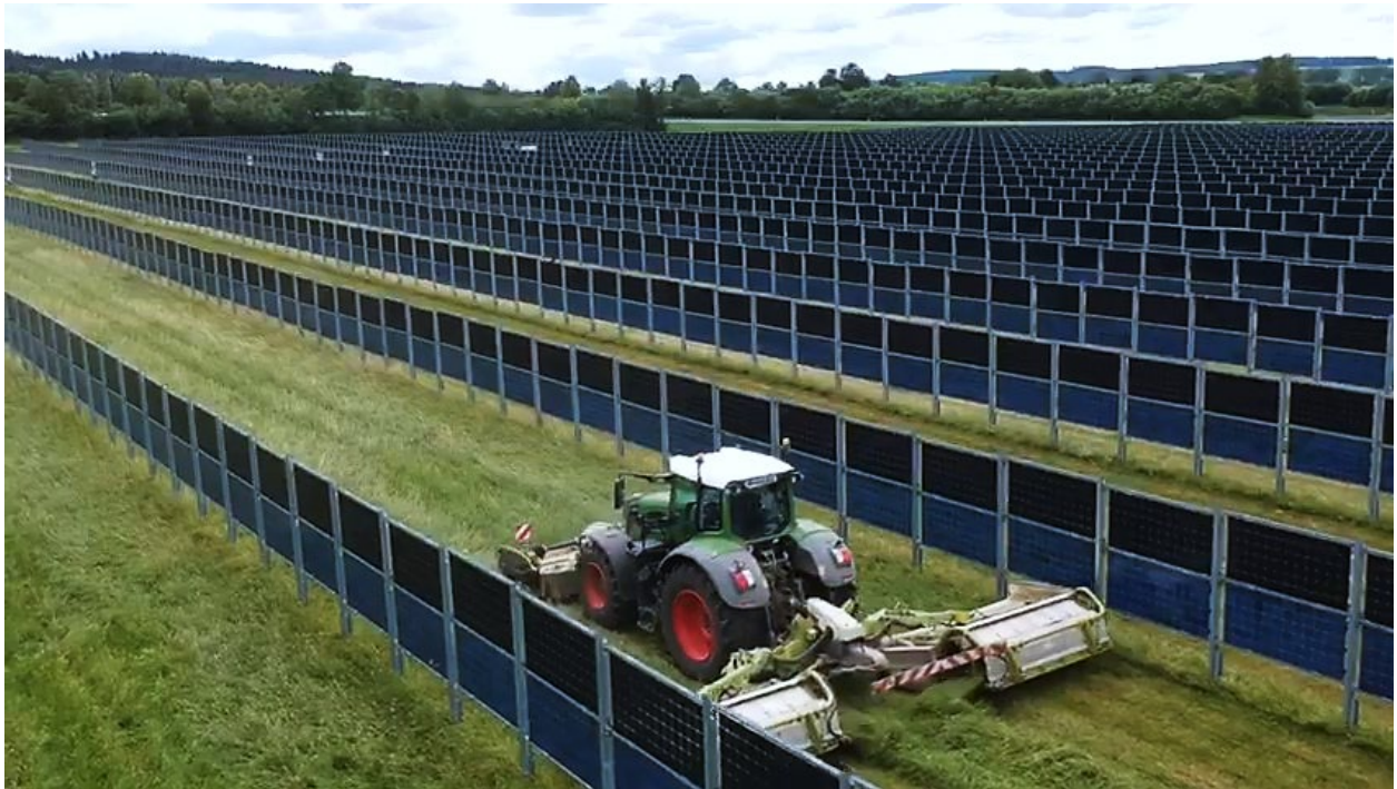
Figure S-8: Bifacial vertically-installed solar panels: Solar Farm, Donaueschingen, Germany Photo credit: Next2Sun GmbH, Germany, with permission
