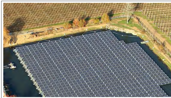
Figure 1.2: Aerial view of a typical agricultural floating solar installation layout over an farming irrigation pond (Pentland, 2011).
