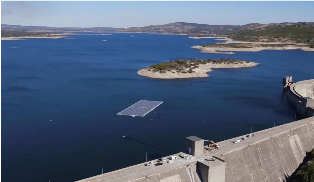
Figure 6. FPV with a pumped hydro “virtual battery” concept. (Copyright EDP S.A., photo by Pixbee).
