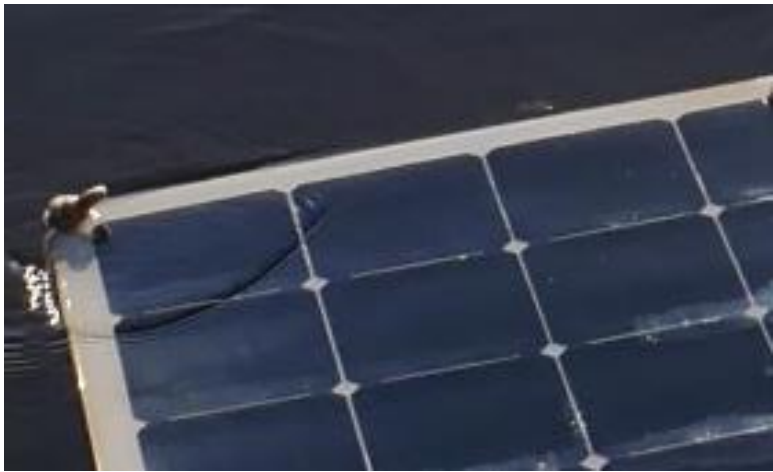
Figure 3.2. Closeup of floating photovoltaic/floatovoltaic (FPV) corner after deployment, showing water coverage from a modest wave (top left).
