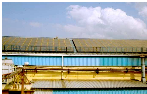
297 m 2 Solor air heating system at TI cycles in Ambatur Chennai
