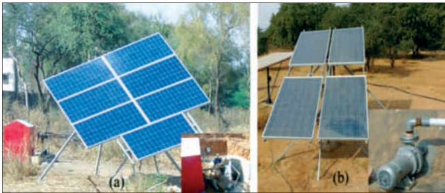
Fig. 1. Solar PV pumping system (a) 1 HP AC pump and (b) 1 HP DC pump
