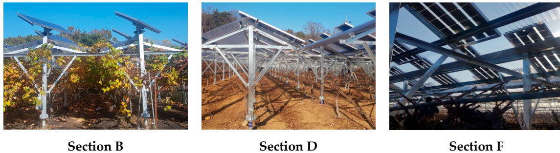
Figure 7. Three types of solar panels. B , normal type; D , bifacial type; F , transparent type.
