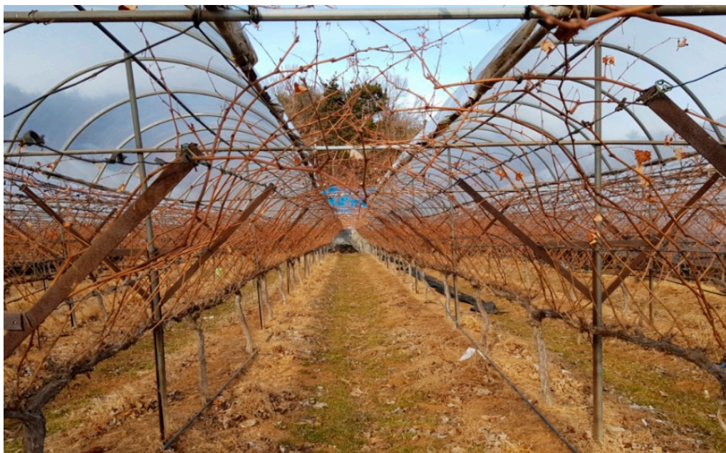
Figure 2. Rain-hit-protection facility in a grape farm.
