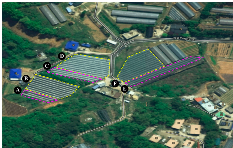
Figure 5. Aerial photo of 3 types of installed panels.
