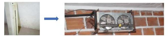
Figure 6-5: Modified Split AC units - locally fabricated fans to blow cool air
