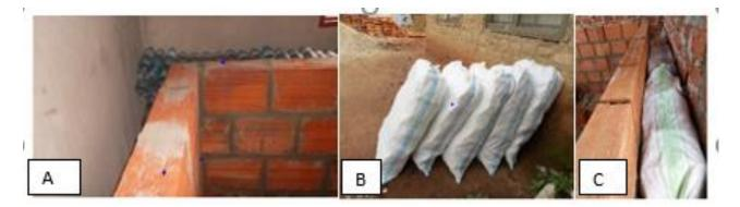
Figure 6-1: A- Insulation used in the 1<sup>st</sup> prototype, **B&C**-Insulation board used in second prototype
