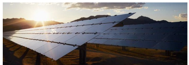
Fig. 2. Photovoltaic park of Sarnia, in Canada. Source: [12].
