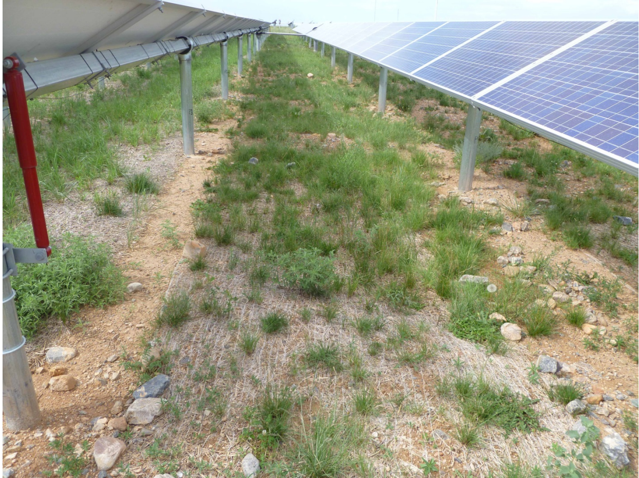
Photograph 10. NWTC tracker arrays arranged in N-S rows that allow sun to reach the ground. Shading from ca. \frac{1}{4} to slightly more than \frac{1}{2} ground surface. The shaded area varies throughout the day. View faces south. Photo Credit: Dave Buckner
