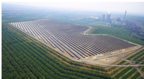
Fig. 6. The 18 MW solar park next to the lignite power plant of Visonta, Hungary.
