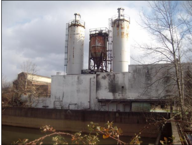
Figure 16. AC&S Chemical Site: Ground view of recommended PV array site
