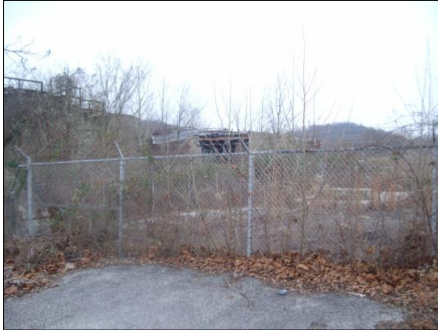
Figure 14. Partially demolished site: Ground view of recommended PV array site
