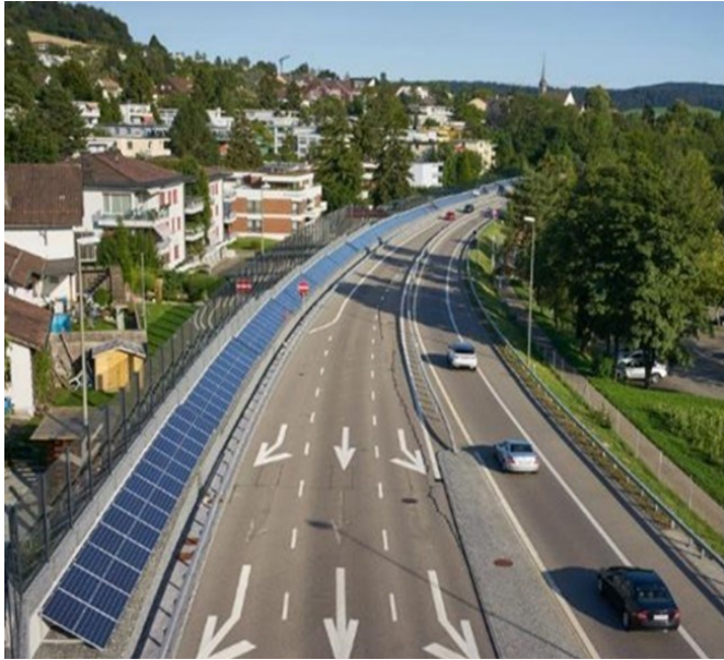
An example PVNB along a highway in Switzerland. Source: TNC Consulting
