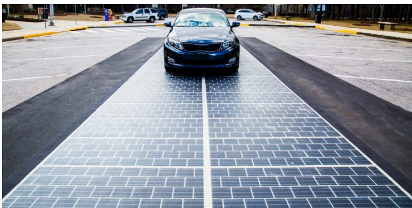
Figure 4: The Wattway drivable solar road surface at the I-85 Visitor Information Center along The Ray (Source: The Ray)
