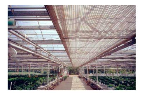
An energy curtain can significantly reduce nighttime heat loss from a greenhouse. Photo: John Bartok, Jr., University of Connecticut
