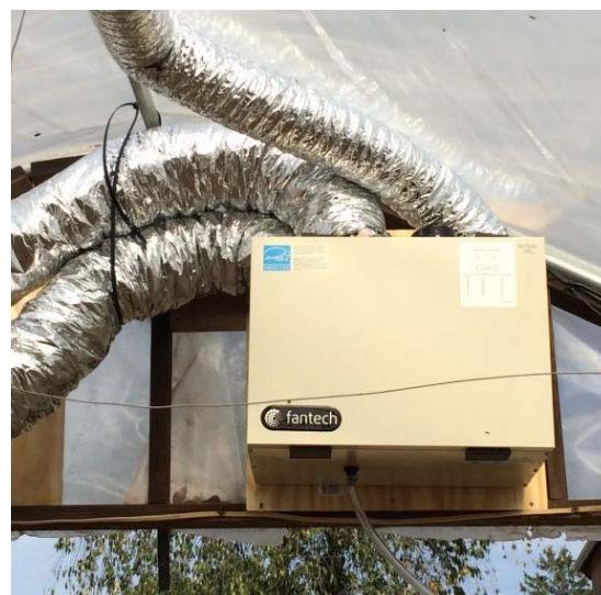
The 106 CFM Fantech heat recovery ventilator installed in the gable of the lower high tunnel (LHT) at New Morning Farm. Photo: Chris Lent, NCAT
