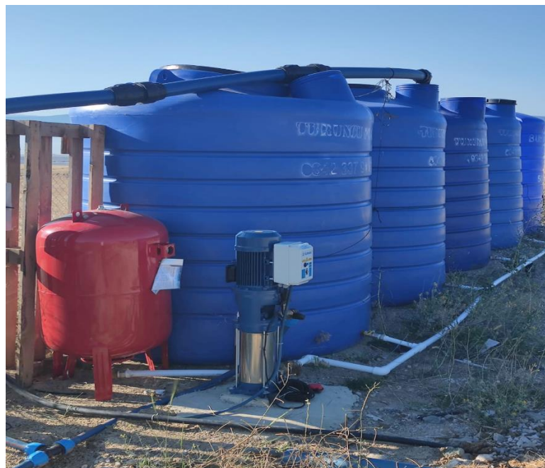
Fig. 7. Second attempt for rainwater harvesting with 25 m 3 tank
