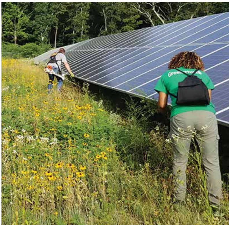
A crew carries out pollinator monitoring and vegetation maintenance at the 1 MW solar array installed by the Sisters of St. Joseph at their campus in Brentwood, NY. © Rusty Schmidt
