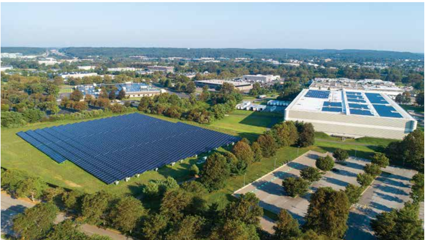
As part of their global citizenship and sustainability efforts, Estee Lauder Companies installed 2 MW of rooftop and ground mounted solar at their campus in Melville, NY. The array provides 100% of the electricity for their office. © EmPower Solar
