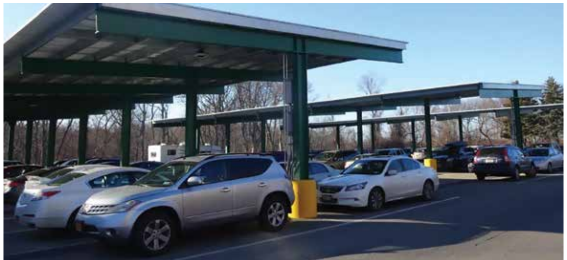
Solar canopies cover parking at the Northport VA Medical Center. © Sunshine Plus Solar
