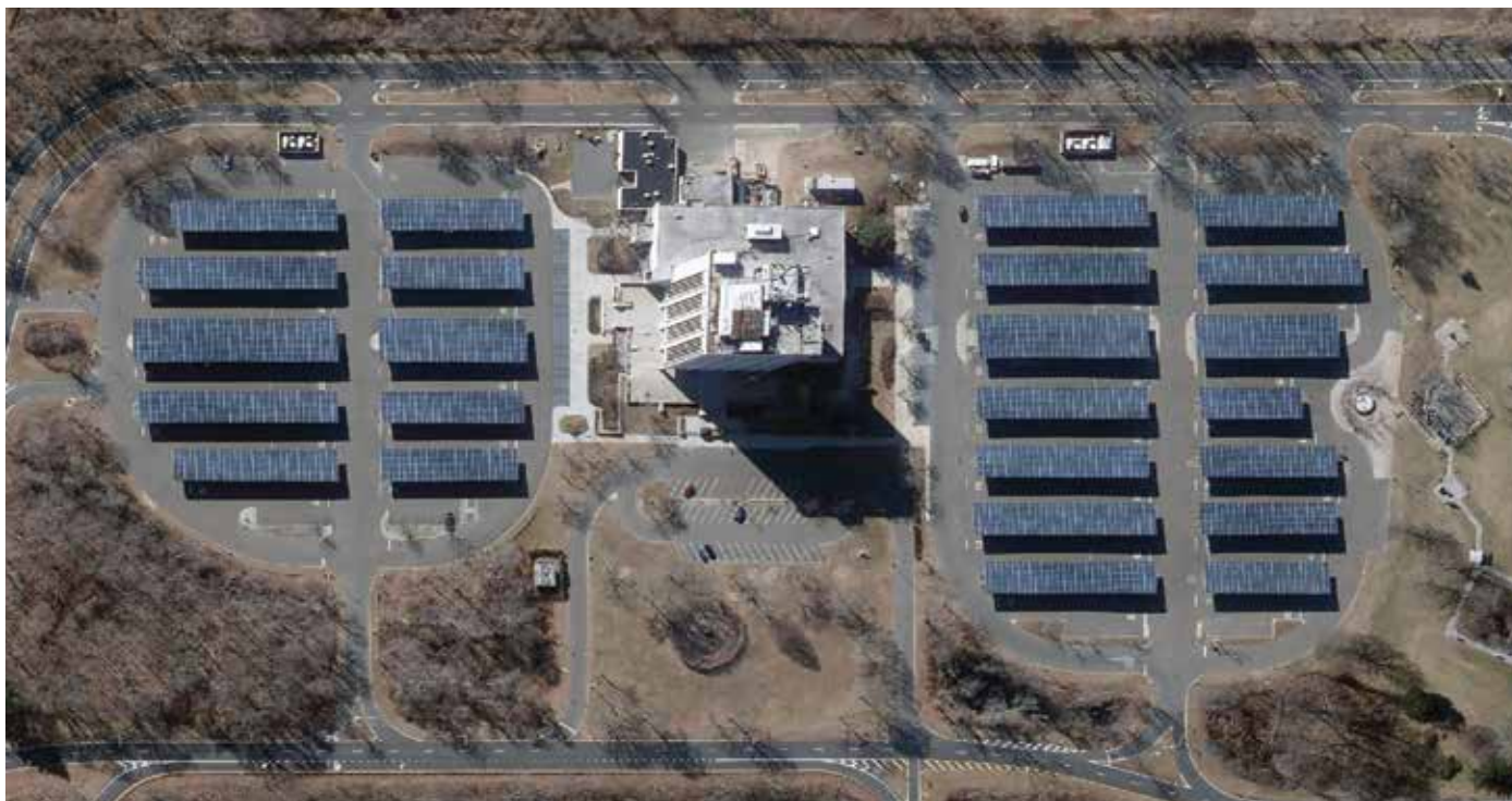
Aerial view of the 1,750 kW solar array in the parking lot of Suffolk County's H. Lee Dennison Building in Hauppauge. Suffolk County has installed solar arrays at six county parking lots and on buildings at seven county facilities. © Suffolk County Economic Development and Planning Department
