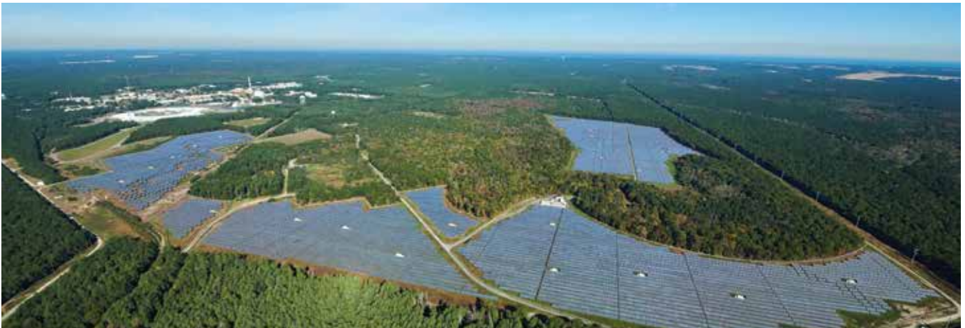
Long Island Solar Farm at Brookhaven National Laboratory © Long Island Power Authority
