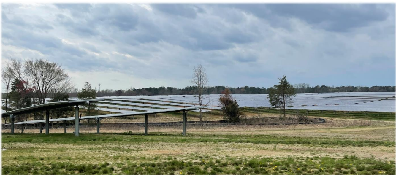
Figure 1. Briel Solar Facility, Henrico County, VA
